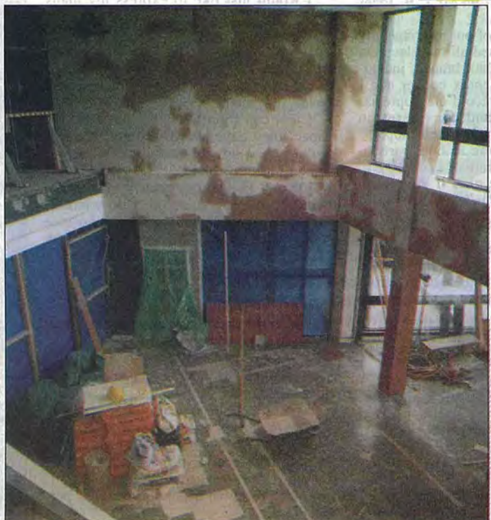
Reception area – during and after refurbishment.
