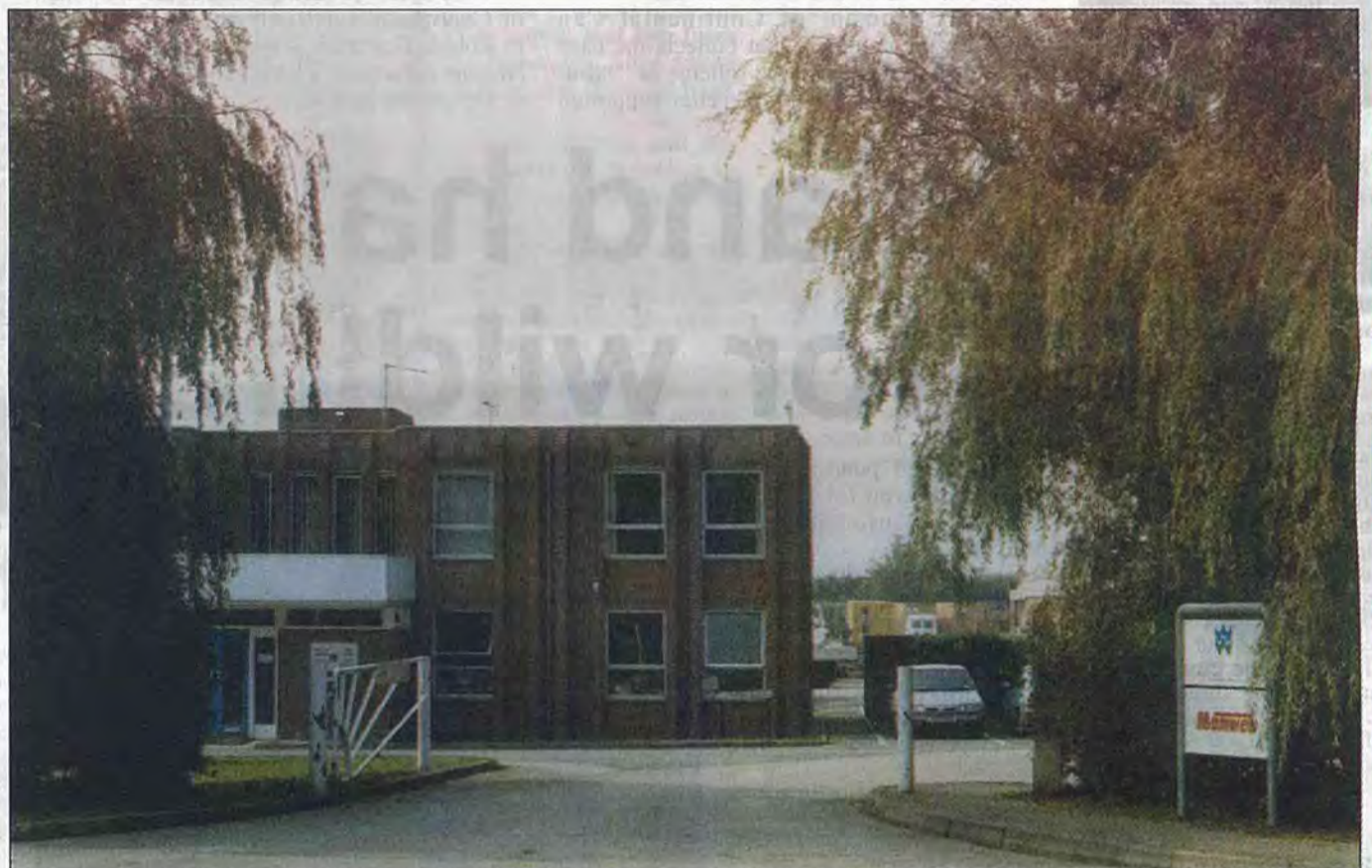
The shared depot at Glan Conwy.
